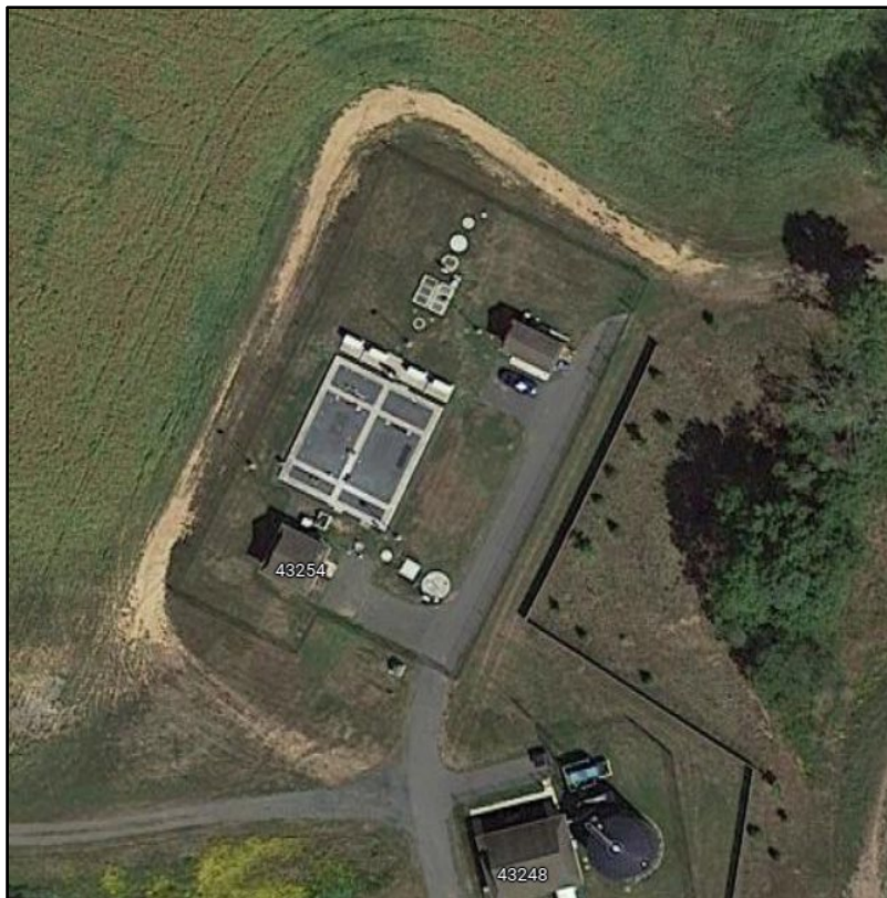
Aerial Photo of the existing Elysian Wastewater Treatment Plant
