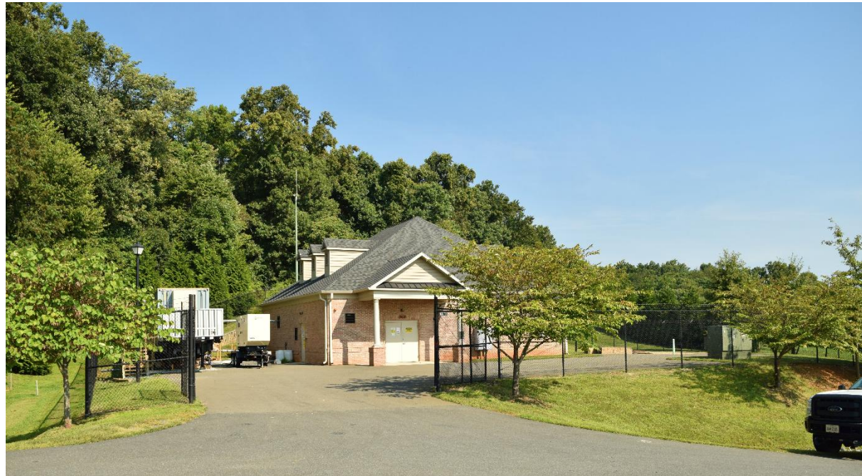
Existing Water Treatment Building
