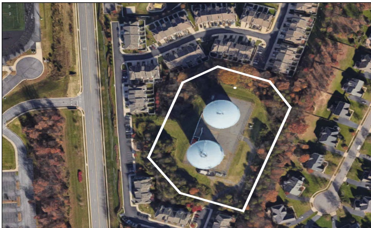
Photo of the existing Brambleton Facility (Tank 2 towards the bottom of the page)
