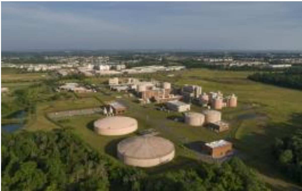
Photo of the existing Broad Run Water Reclamation Facility
