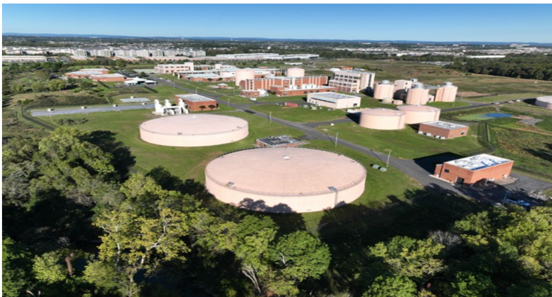
Photo of the existing Broad Run Water Reclamation Facility
