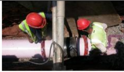
PVC Pipe Installation
