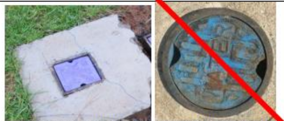
Reclaimed Water Valve Cover vs. Potable Water Valve Cover. Use square shape in roadways.
