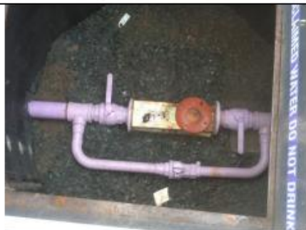
Meter Pit With Low Rise Setter
