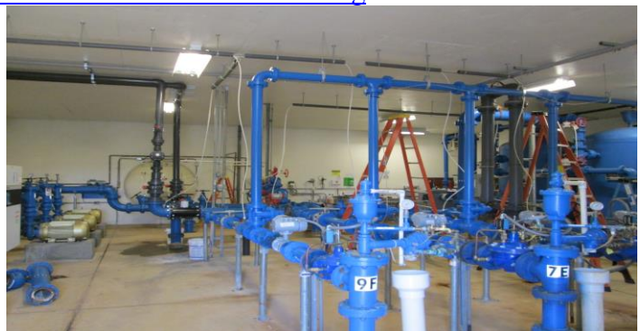
Photo of the existing Selma Water Treatment Plant
