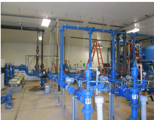
Photos of existing Selma Water Plant
