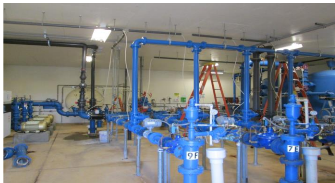
Photo of the existing Selma Water Treatment Plant
